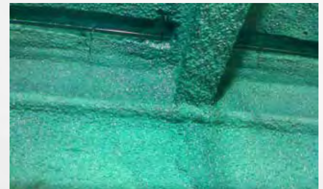
ABC Green applied to asbestos containing fireproofing on structural steel beams
