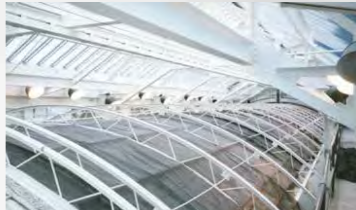
A view from inside the attic after LBC was applied
